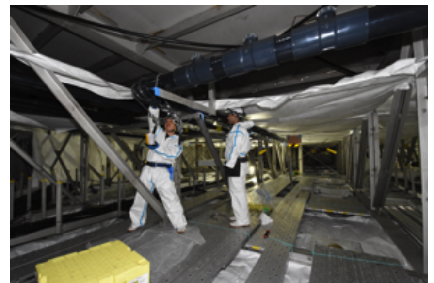
Install new water pipe
