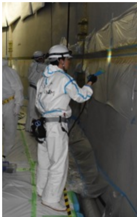
Seal whole welding lines
